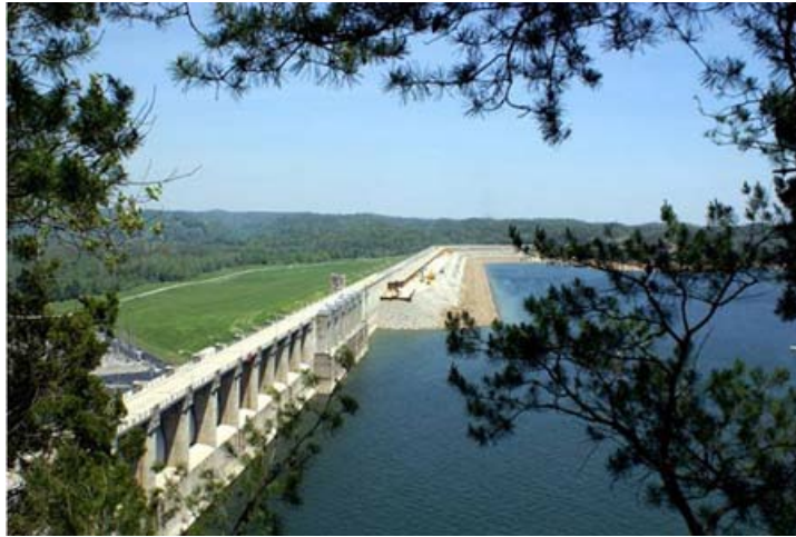
East Lake Dam
